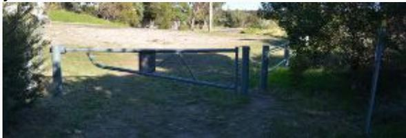
Metal bollard pinch points at edge of carpark, beside gate. The gap between the bollards is 48cm they are 85cm high.
