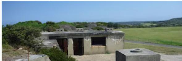
This World War Two bunker is near the Westpac Helicopter Shed. This bunker consists of sheltered concrete ammunition storage rooms below, and a circular gun base above, with surrounding coastal views. There are rusted and damaged parts, so take care when exploring.
