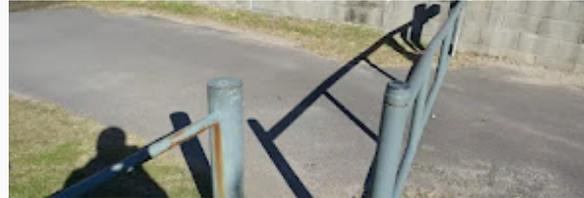
Metal bollard pinch points at edge of carpark, beside gate. The gap between the bollards is 55cm they are 85cm high.
