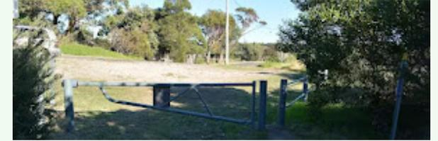
Metal bollard pinch points at edge of carpark, beside gate. The gap between the bollards is 48cm they are 85cm high.
