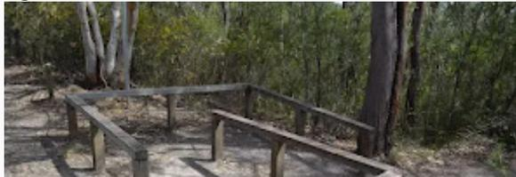
Timber guards. Minimum width between the guards is 1.2m (maximum is 1.38m).
