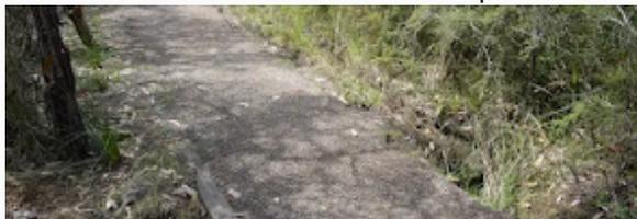
A trip hazard on the path. Potential fall of the the side with no guards. The path is 1.1m wide and the fall is 40cm on either side of the path.
